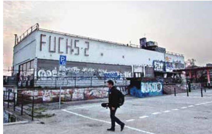
WINTER STADIUM RESTAURANT AT ŠTVANICE / Prague, Czech Republic
